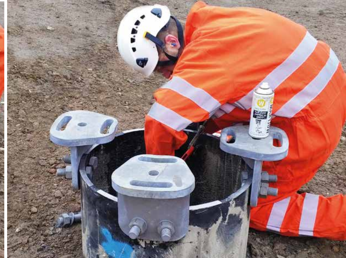
Bolt on Flexi-Pile Cap tabs.
