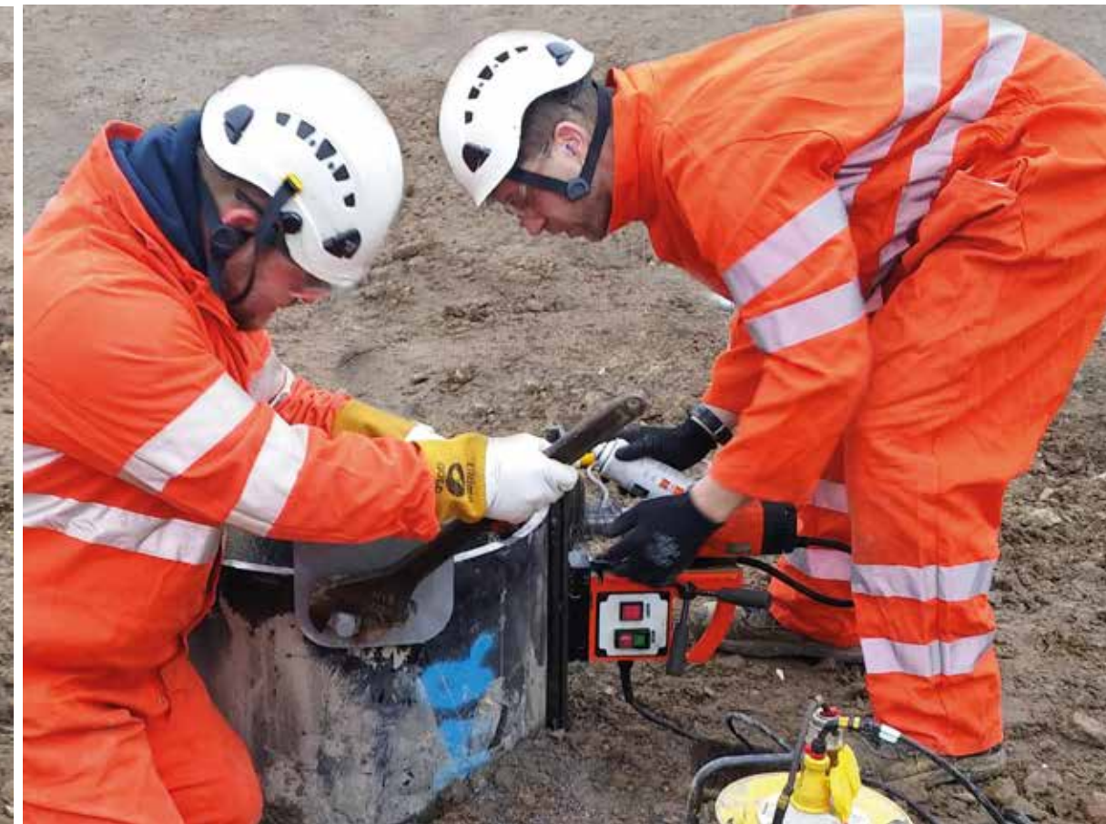
Drill holes using a template.
