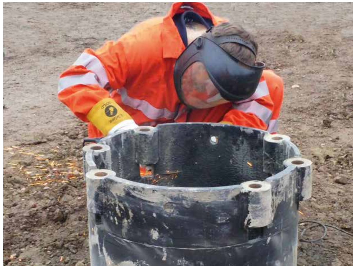
Cut pile to Height.
